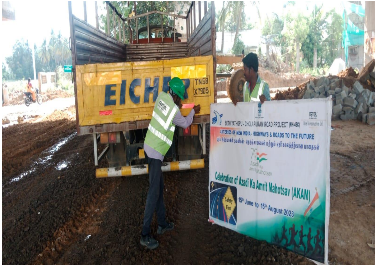
Safety Reflecting stickers pasting at Ch. 117+700
